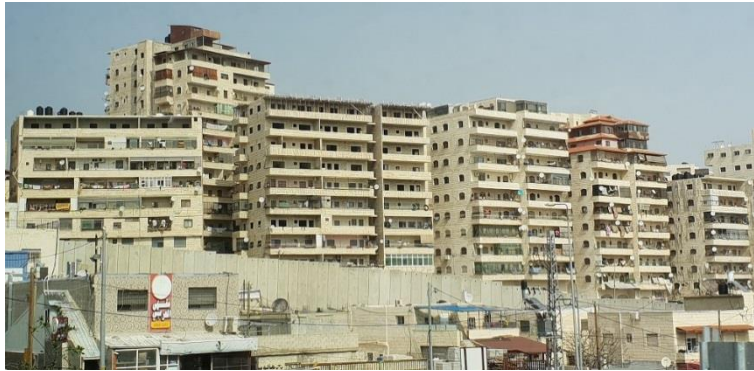
Figure 4.1: Ras Khamis buildings – view from the Shu'fat village. Source: Author, February 24, 2019.
