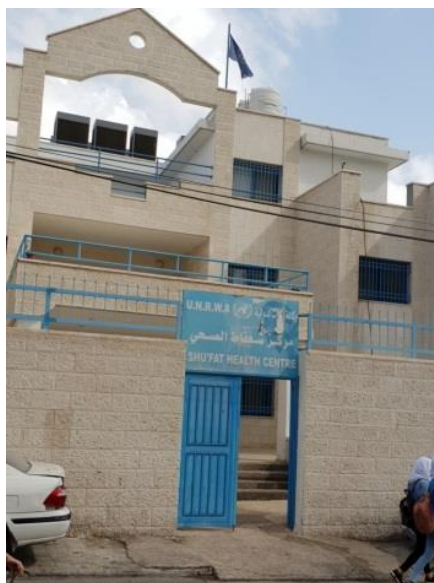
Figure 5.4: UNRWA Health Center – Shu'fat Refugee Camp. Source: Author, October 17, 2018.
